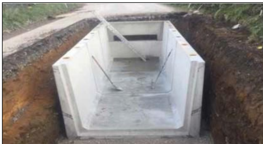
Figure 2-4: Typical Joint Bay Installation (Source: Eirgrid)
